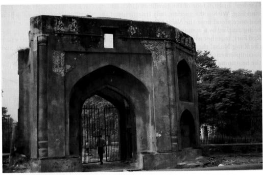
Fig.~4 The Gateway of the Roshanara Bagh showing its condition in 1997 with some loss of encaustic work
